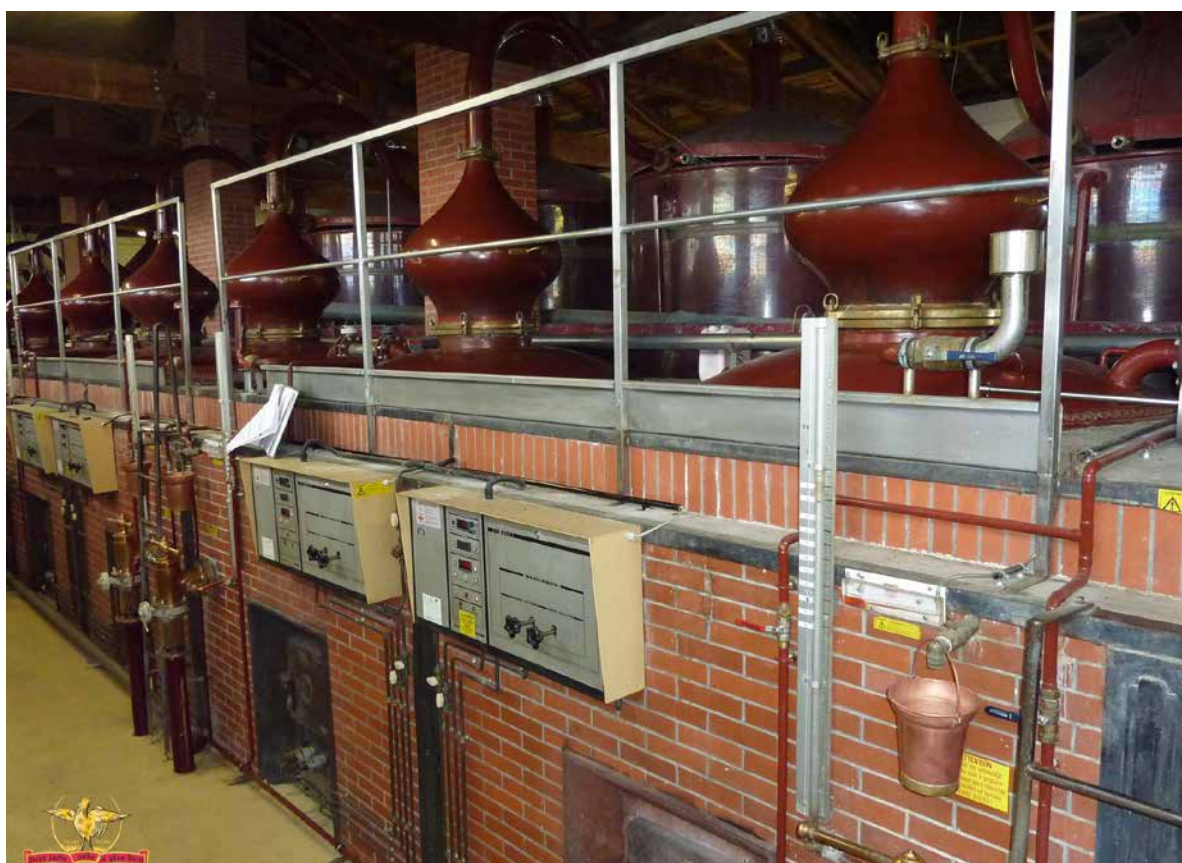
MAISON THE FILLIOUX FAMILY (CREDIT: VINOPURO.COM). LEFT, FILLIOUX CHARENTAIS ALEMBIC STILLS.
